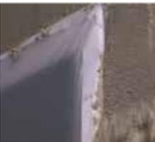
6. Remove sheeting which will pull out perforated portion of foam
